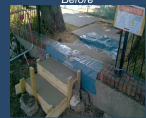
After (work in progress)
