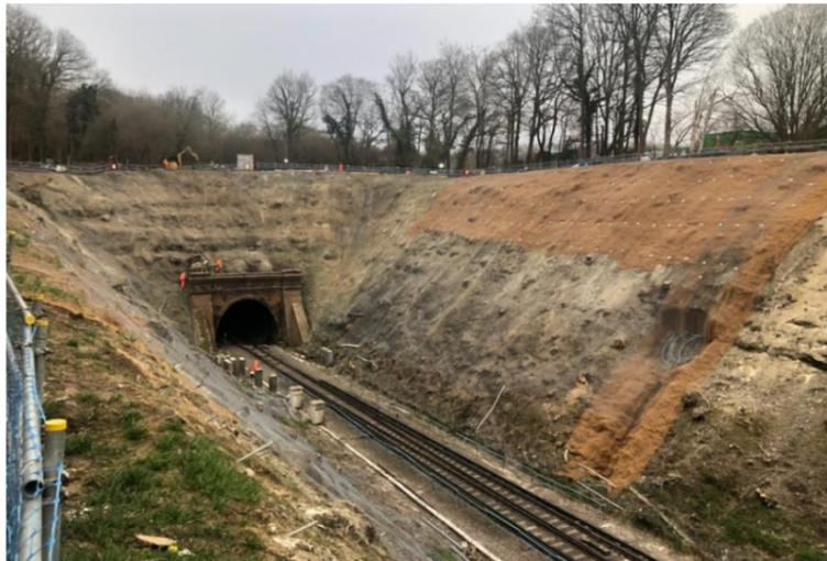
The ground type varies between rock and soil at this location, so in order to provide the best solution, an active soil nailing and netting fix is being implemented on the top half of the cutting with a passive drape netting on the lower half.
