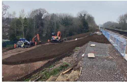
Meanwhile, south embankment works are cut/regrade, installation of badger netting, relay trough and provision of a walkway, South embankment also has a Redi-Rock wall installed at the toe.
